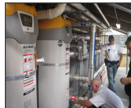
Our technician, Dave, installing HydroCare at UC Davis
